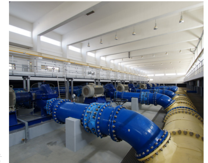
Sanitation for the city of Al Ain. United Arab Emirates.
