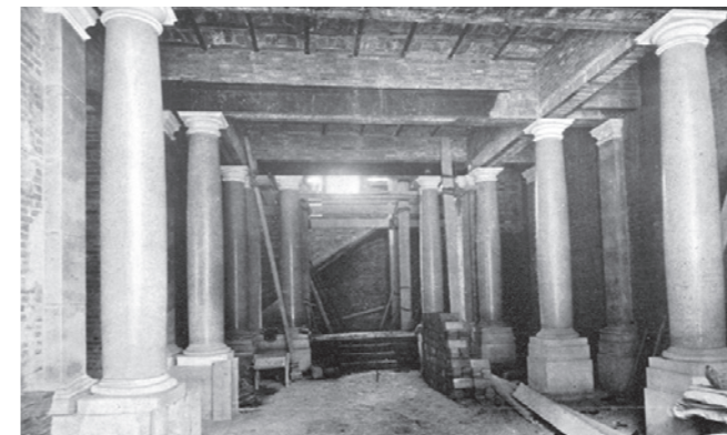
Construction of FCC Head Office on Calle Balmes. Barcelona.
