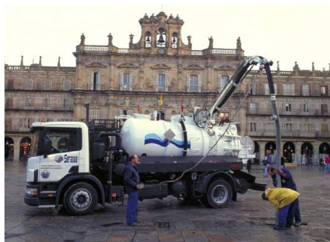
Drains cleaning. Salamanca.
