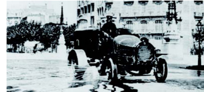
First motorised street cleaning vehicle. Barcelona.
