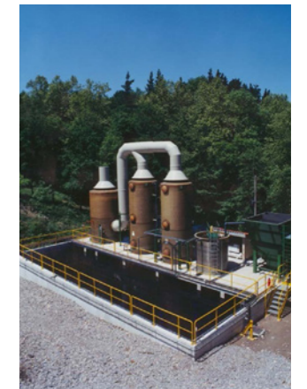
San Marcos leachates treatment plant. Guipúzcoa.
