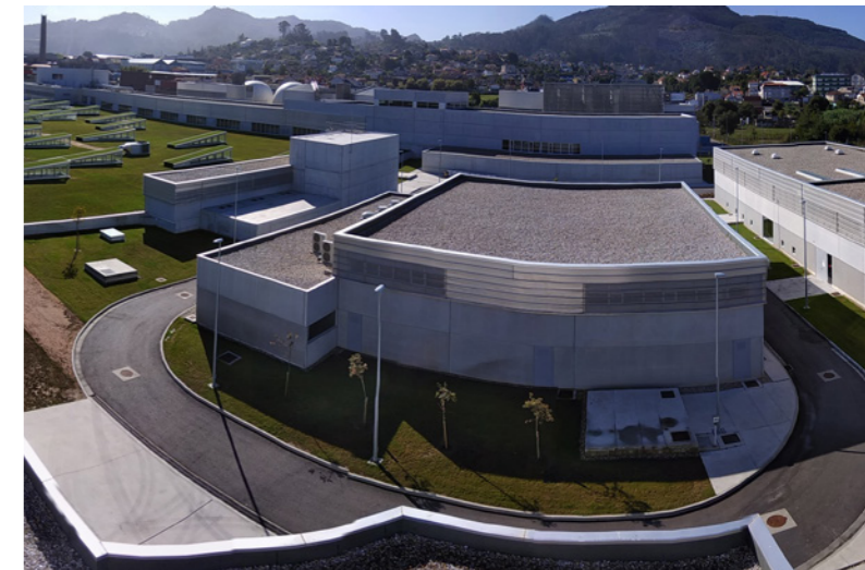
Drinking water treatment plant. Vigo.
