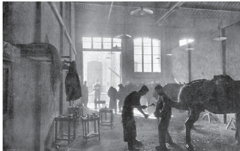
Blacksmithing workshop. Barcelona.
