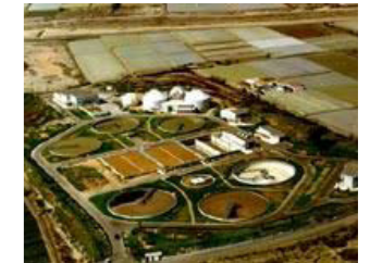
Costacabana waste water treatment plant. Almeria.
