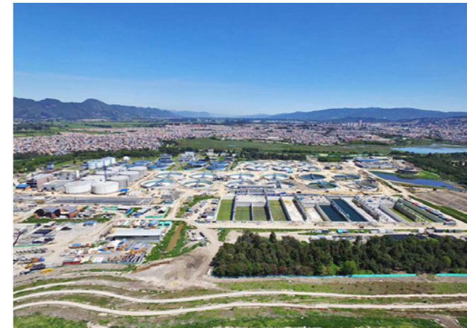
El Salitre waste water treatment plant. Colombia.
