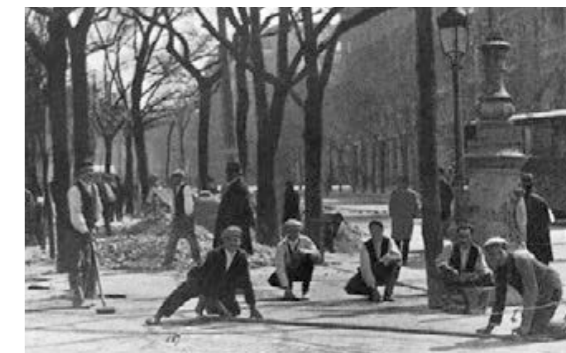
Cement pavements being laid on Calle Alcalá. Madrid.
