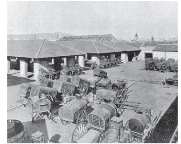
FCC vehicle yard on the Port Montjuic highway. Barcelona.
