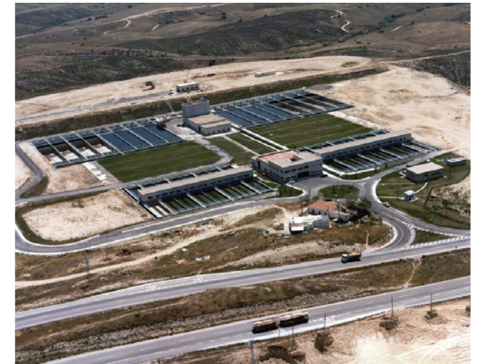
El Atazar waste water treatment plant. Madrid.
