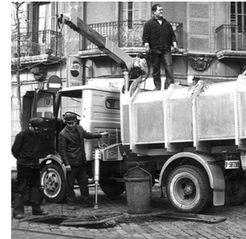
Sewer cleaning equipment. Barcelona.
