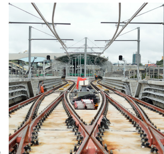
Line 2 of the Panama Metro.
