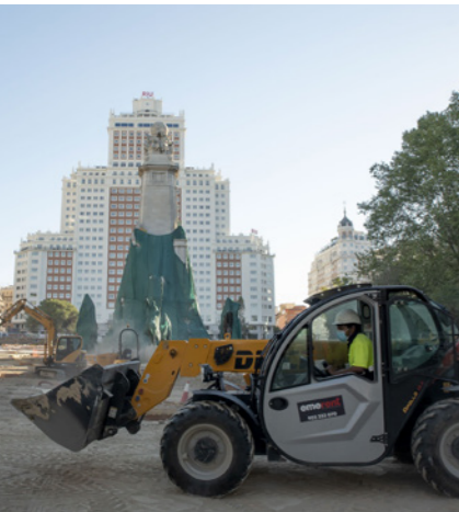
Construction work on the Plaza de España, Madrid.
