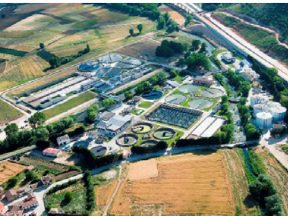
Burgos water treatment plant.
