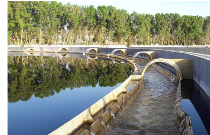
Arana treatment plant in Mecca, Saudi Arabia.
