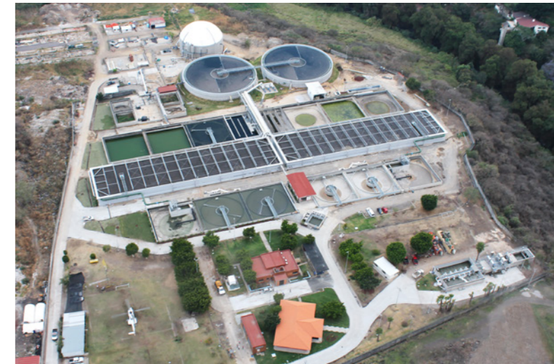
Cuernavaca Waste Water Treatment Plant in Morelos, Mexico City.
