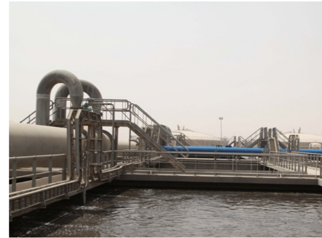
New Cairo treatment plant. Egypt.
