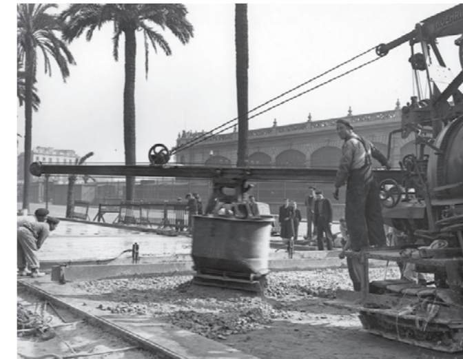
Urban development of Calle Colón with vibrated concrete. Barcelona.
