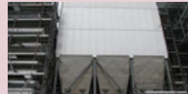
Dry offgas cleaning and pollution control system with activated adsorption, bag filter and NOx reduction clean emissions.
