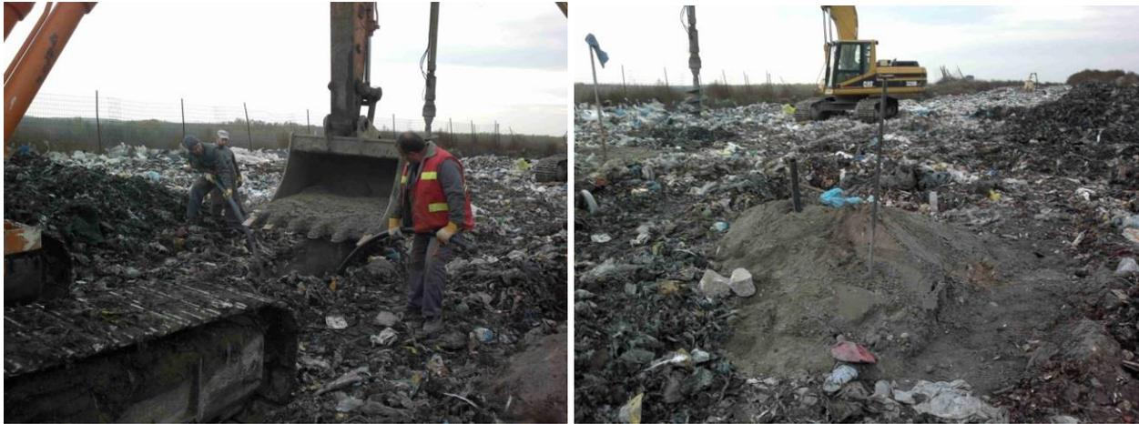
Figure 4. Construction of vertical heat exchanger wells.
