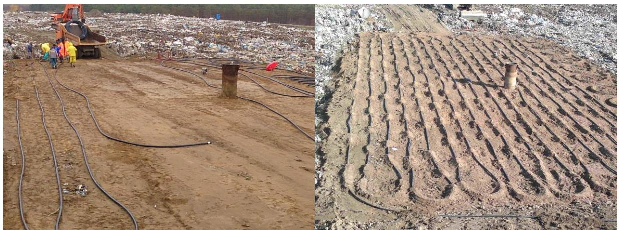
Figure 3. Construction of the “ladyfinger” and the “Slinky” types of heat exchanger pipelines.
