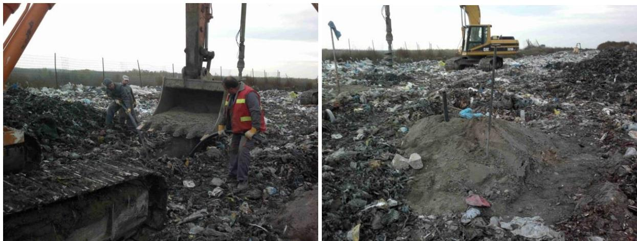
Figure 4. Construction of vertical heat exchanger wells.
