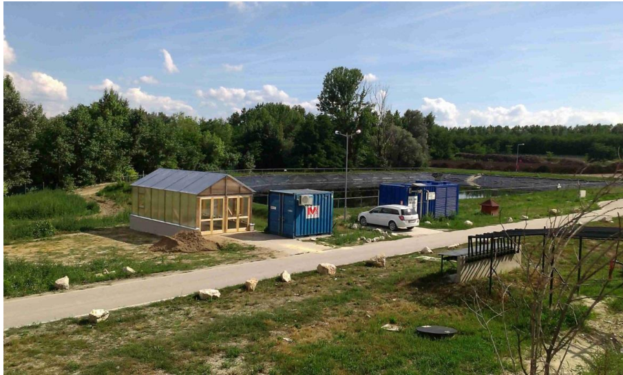
Figure 7. The built greenhouse, the container functioning as engine-house and the leachate pond.
